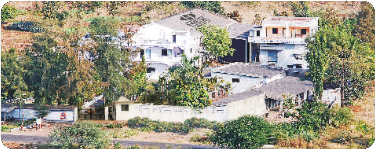
HEX Factory situated near Vapi, Gujarat.
